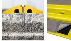
Position speed bump where you would like to install it. Using its molded holes as a template, mark the location of each hole on the roadway's surface.
